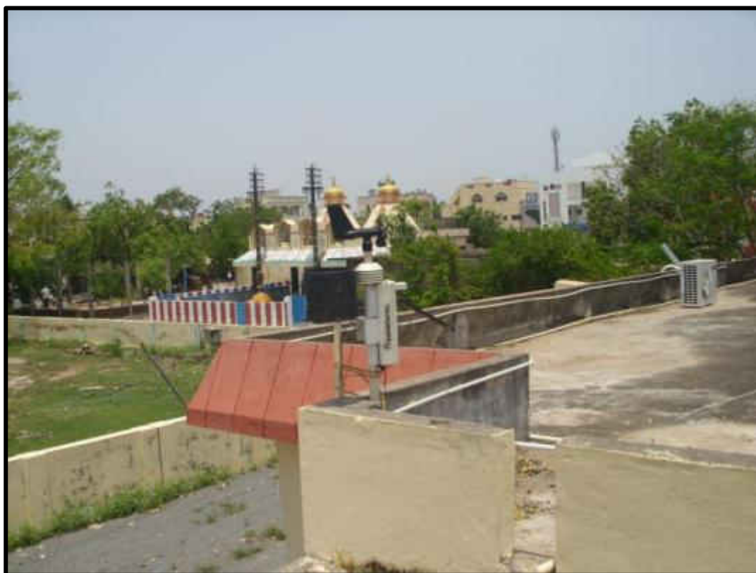
Figure 5-1 Automatic weather station installed at Thulluru
